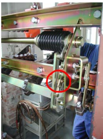
OFF position break lever (back view)
