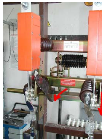
Switching the device off without using the operating drive (front view)
